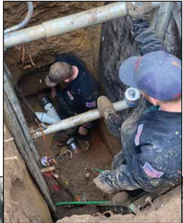
Below: 14 ft hole to repair broken sewer line
