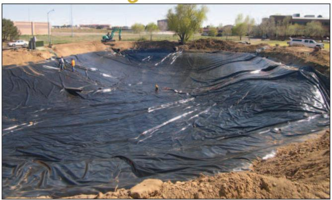
Large pond along South Xanadu Way at the #5 tee box gets a new liner. Above: looking south at same pond. Note how small the workers are in this large pond. It will be the major source of irrigation water. Below: Dry creek bed along which pipes to transfer water are being laid.
